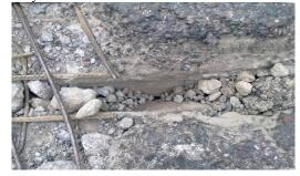
FIGURE 2. The destruction of hinge seam
